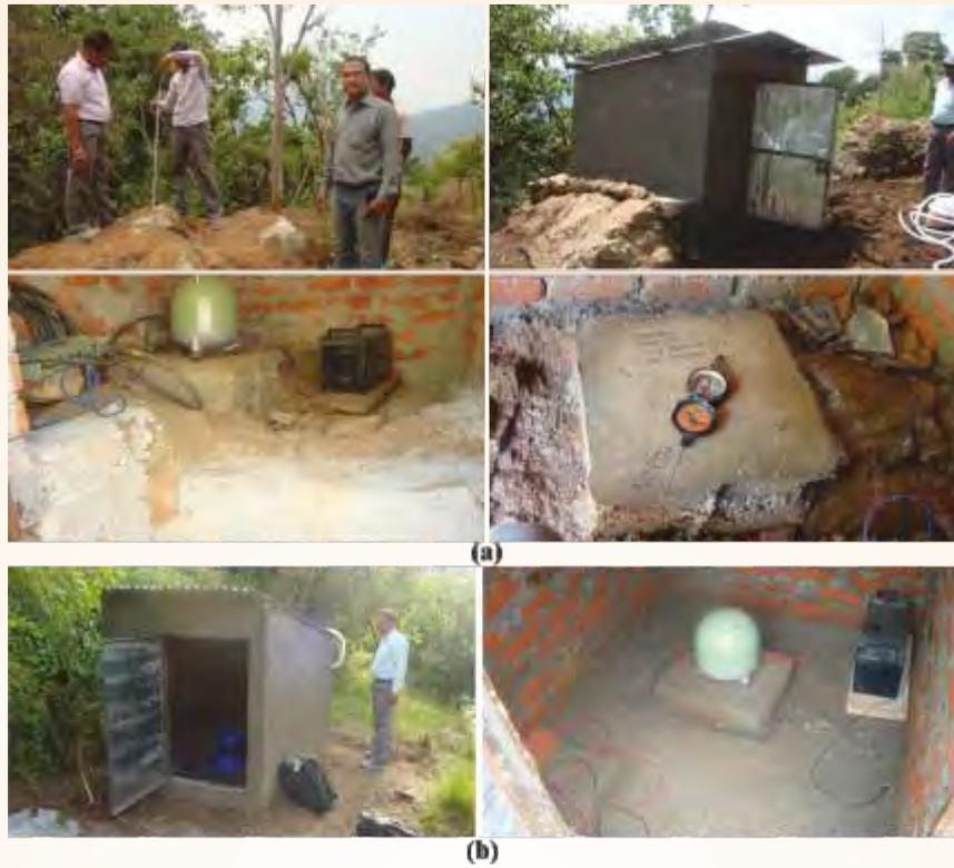
**Fig. 57:** Photographs during seismological Pit and Hut construction at (a) Matela village and (b) Champawat, Kumaun Himalaya.
