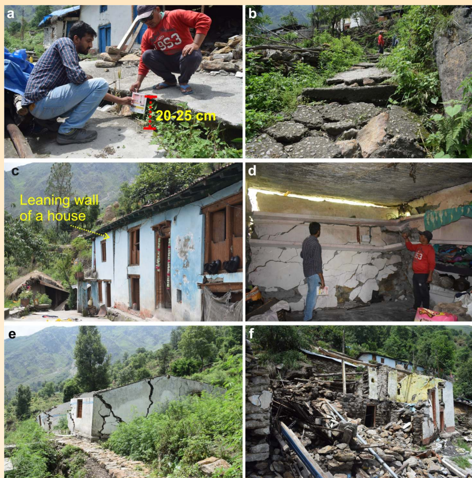
Fig. 49: Photographs showing subsidence-induced indications as observed at various places in Dar village (a) cracks in the ground, (b) displaced stairs, (c) leaning wall of a house, (d) cracks in the walls of a house, (e) collapsed building of a primary school and (f) a collapsed house.
