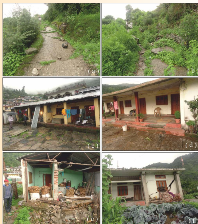
Fig. 48: Footpaths and houses affected by landslides at Barsu which result from toe cutting by Swari Gad a tributary of Bhagirathi River.
